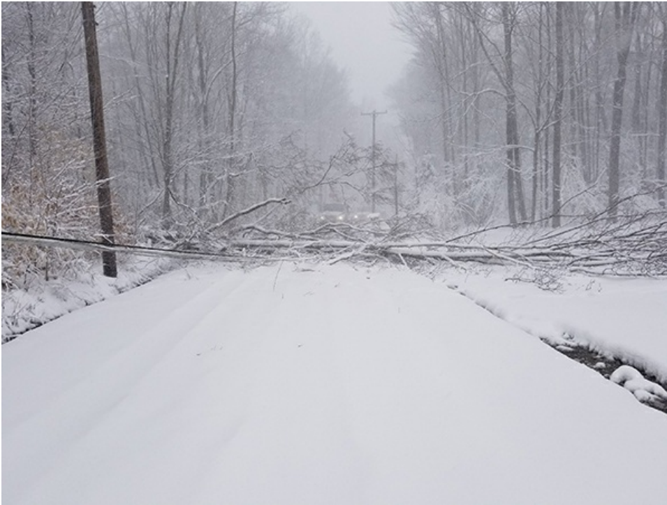
A scene of storm damage from Elmhurst, Pennsylvania in Lackawanna County.
